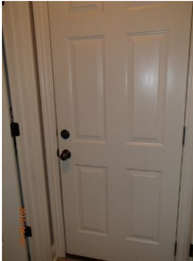
Exterior Door Condition
