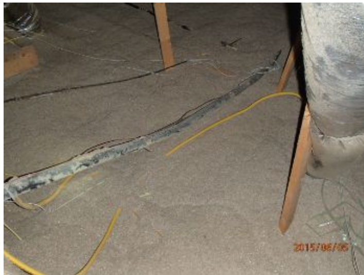
Attic Insulation Condition
